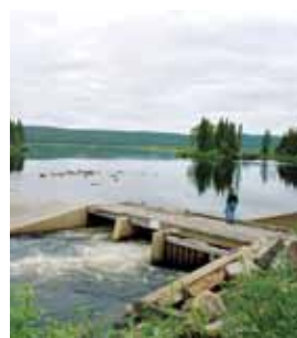
Water Control Structure
