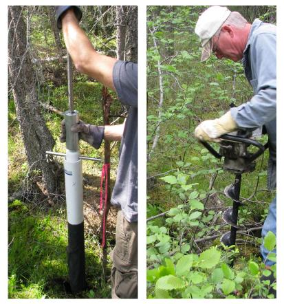
Figure 3. View of the two tools used to install the monitoring wells. A typical pounding tool was used to drive the well tubes into place (left). The job was made easier when a gas-powered auger was used to first create a pilot hole (right).
