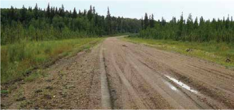
Soft road surface and rutting can be caused by blockage of flow.
