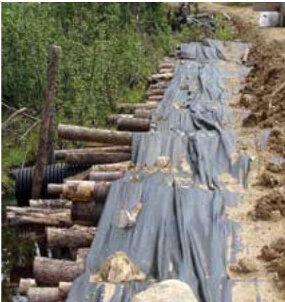
Extending geotextile helps prevent sediment from entering waterways.
