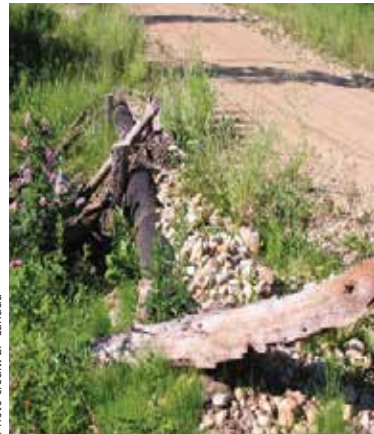
Curb logs can help contain road fill.
