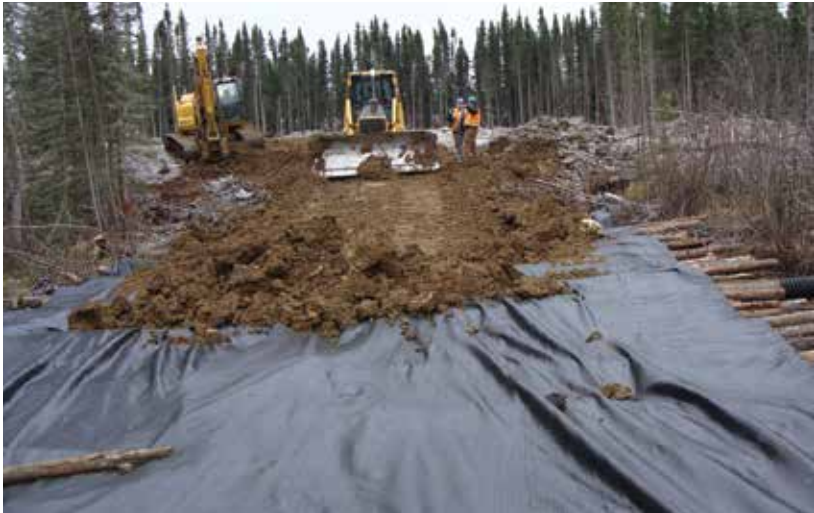
Geotextile used as a separation layer.
