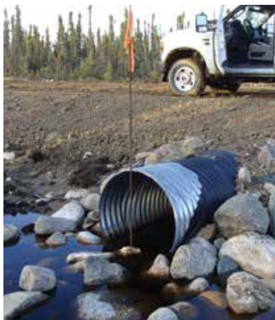
Culverts should be embedded.
