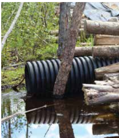
Example of culvert used in combination with corduroy.
