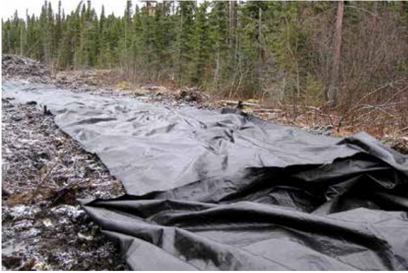
Geotextile placed over uneven road surface.
